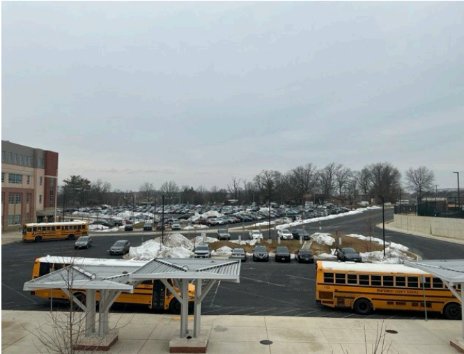
31 - FRONT PARKING LOT
