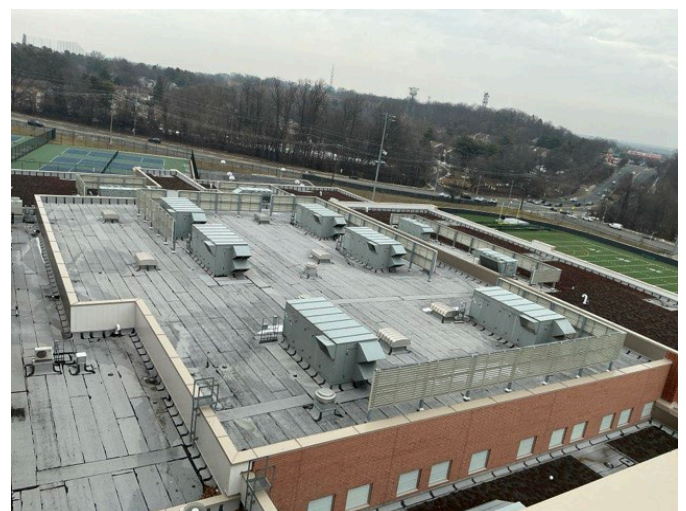
18 - BITUMEN ROOF / ROOFTOP UNITS
