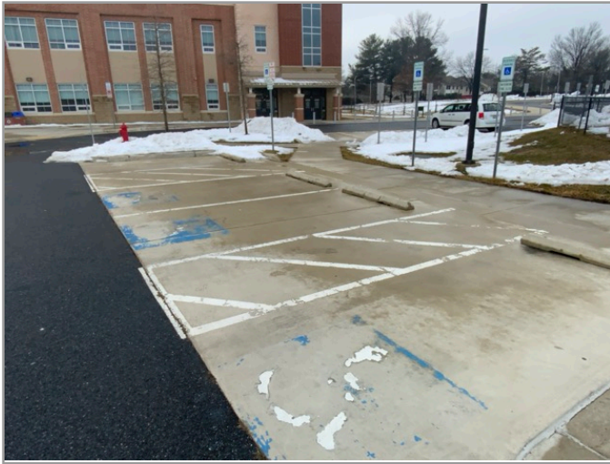
OVERVIEW OF ACCESSIBLE PARKING AREA
