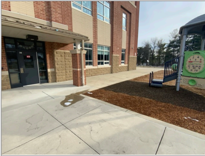
ACCESSIBLE ROUTE TO PLAYGROUND
